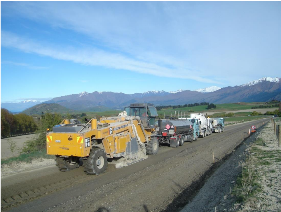
Figure 4.12: Foamed bitumen stabilisation construction train
