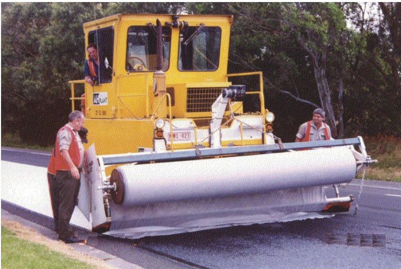
Figure 4.18: Applying a geosynthetic before sealing
