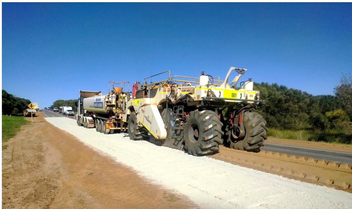
Figure 4.8: Cement stabilisation construction
