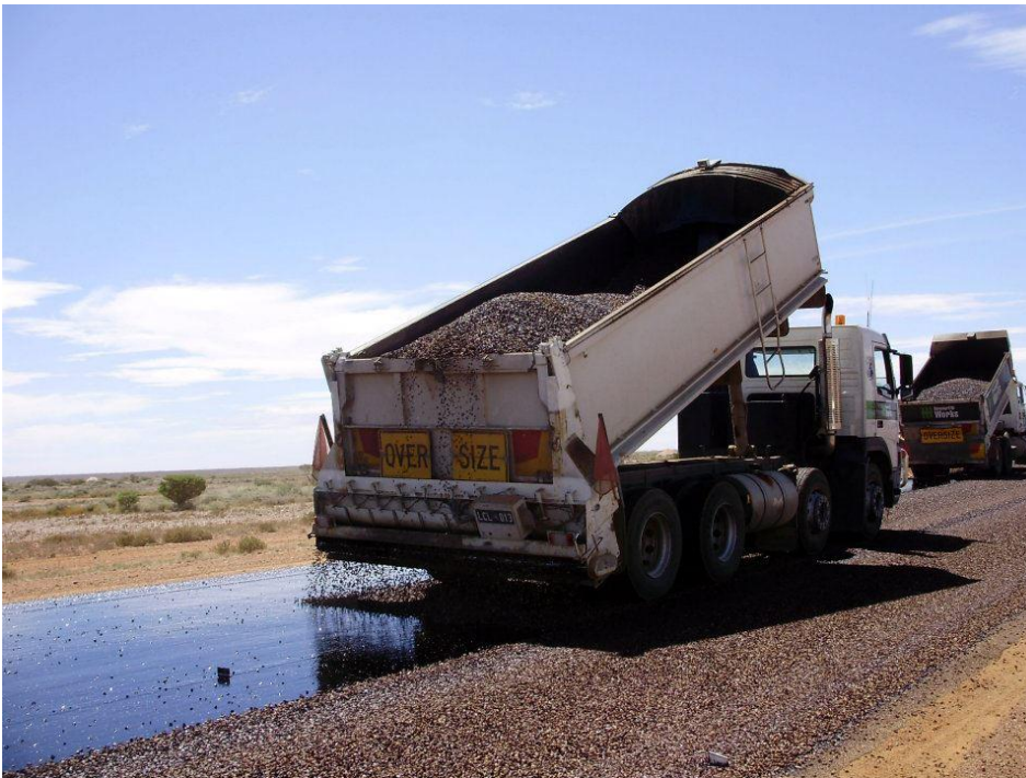
Figure 3.4: Sprayed seal construction
