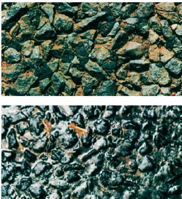
Coarse aggregate seal (top) before and after (bottom) application of a surface enrichment of about 0.7 L/m 2
