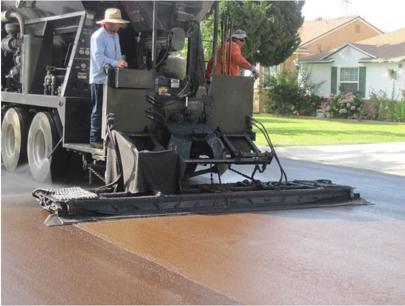
Figure 5.2: Application of a slurry seal
