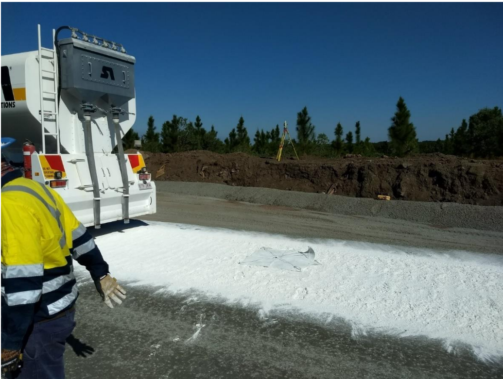
Figure 4.11: Checking lime spread rate during lime stabilisation
