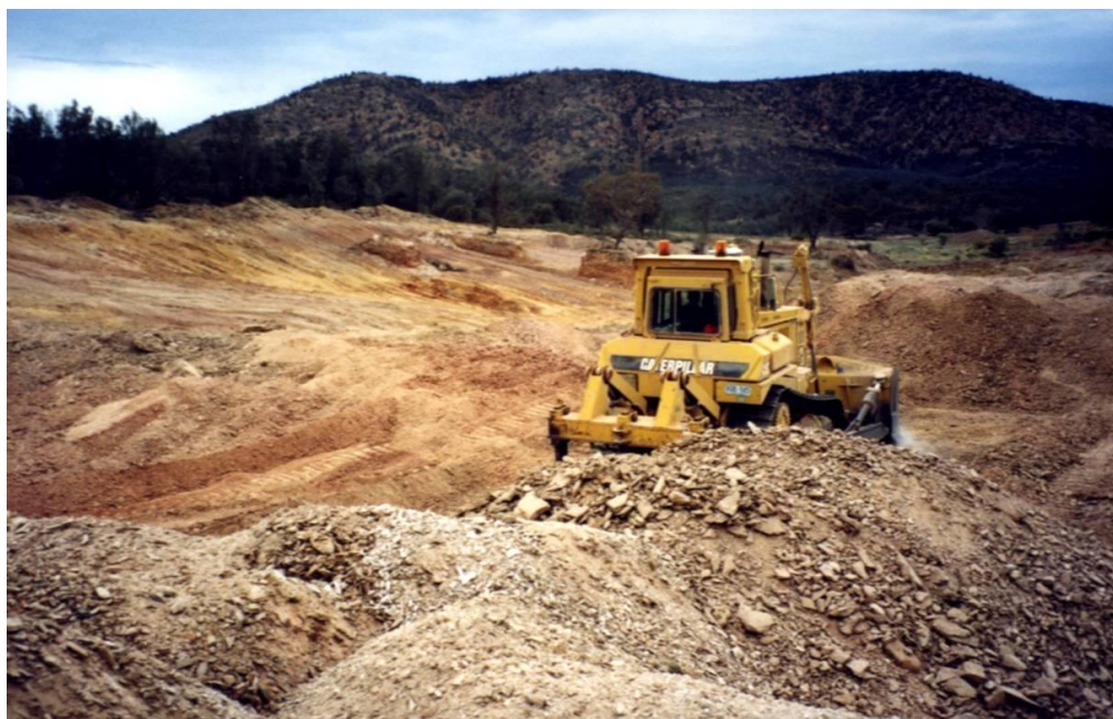
Figure 4.1: Dozer working a local borrow pit
