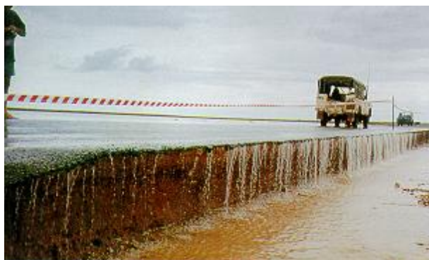
Figure B 4: Geotextile reinforced seal and shoulder erosion
