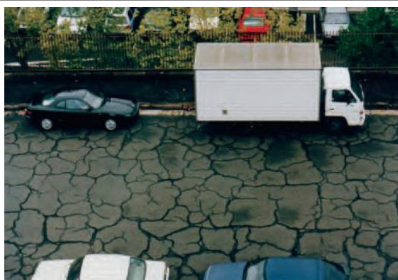
Figure 5.4: Crocodile cracking – closely spaced, interconnected cracks forming scale-like polygons
