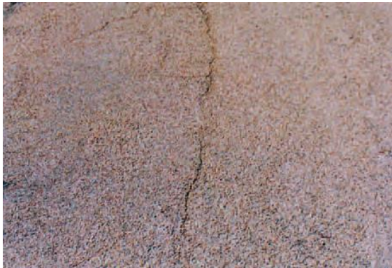
Figure 5.8: Transverse cracking – unconnected crack stretching across the pavement
