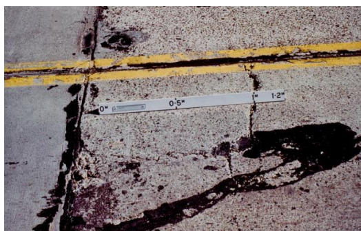
Figure 5.24: Rocking – rocking movement of a slab under traffic
