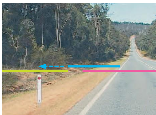
Figure 4.6: A typical road profile with the clear zone extending just beyond the upside of the table drain
