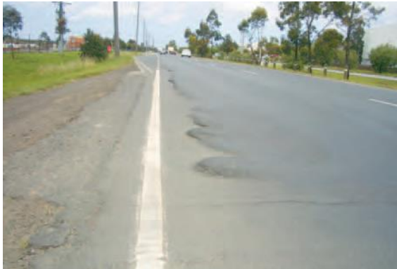
Figure 5.14: Flushing – excess appearance of binder at the pavement surface
