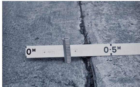
Figure 5.23: Faulting – permanent vertical separation of two slabs at a joint
