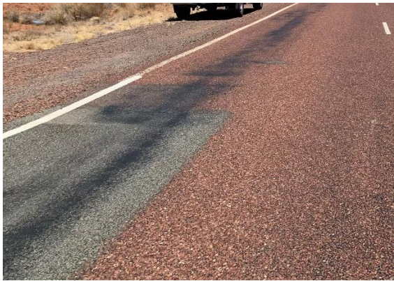
Figure 5.16: Polishing – smooth, potentially shiny, rounded surface aggregates
