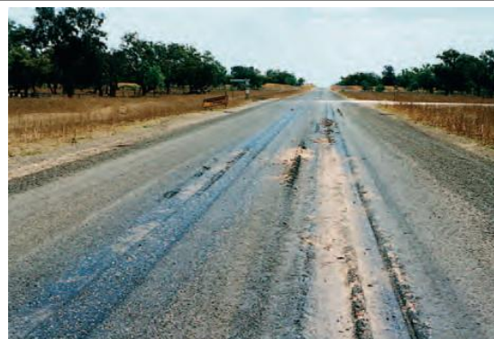
Figure 5.11: Rutting – longitudinal deformation in the wheel path
