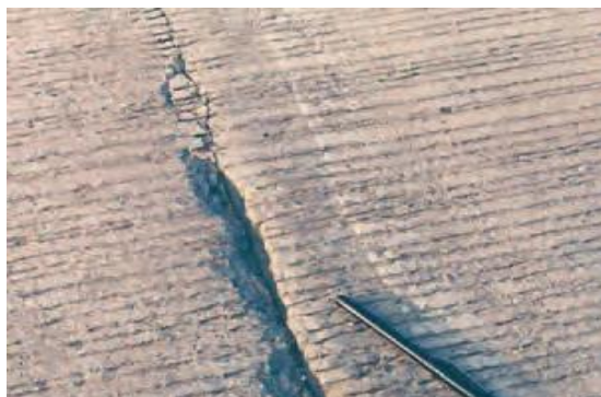
Figure 5.24: Rocking – rocking movement of a slab under traffic
