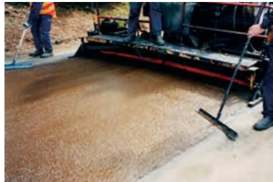
Figure 5.36: Slurry seal
