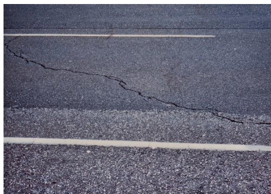
Figure 5.5: Diagonal cracking – unconnected cracking stretching diagonally across the pavement
