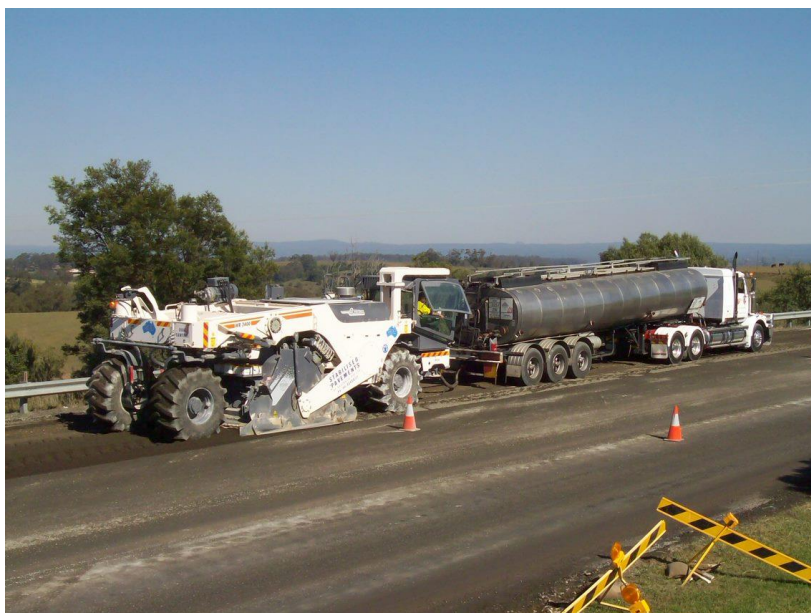
Figure 4.12: In situ stabilisation
