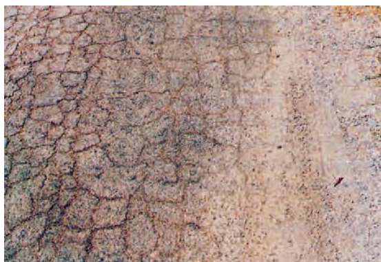
Figure 5.4: Crocodile cracking – closely spaced, interconnected cracks forming scale-like polygons
