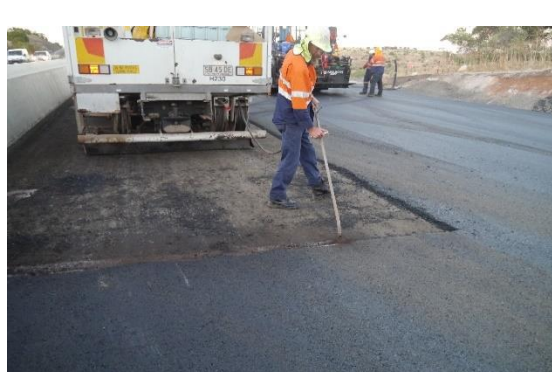
Figure 5.34: Tack coating asphalt patch
