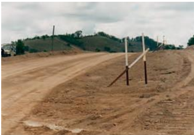
Figure 4.10: Setting out roadworks in cuttings and on fill
