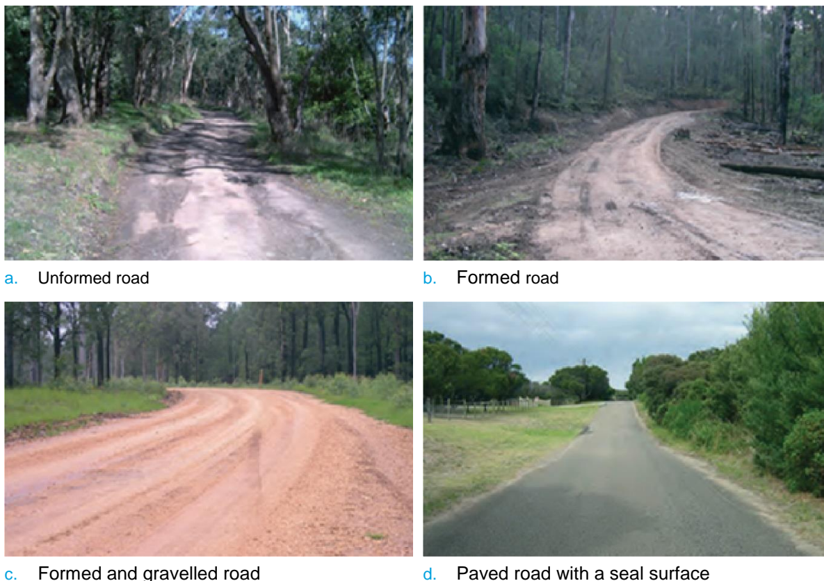
Figure 3.1: Stages of road construction
