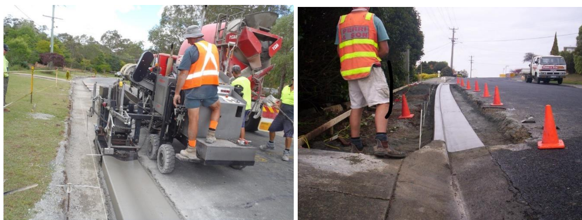
Figure 4.8: Construction of kerb and channel
