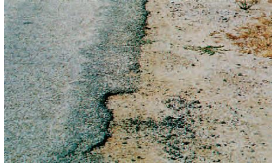
Figure 5.21: Pothole – rough, bowl-shaped pits extending through the wearing course and into the layers below
