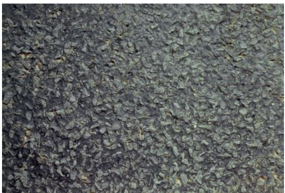
Figure 5.16: Polishing – smooth, potentially shiny, rounded surface aggregates
