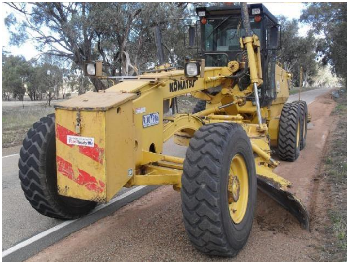
Figure 5.37: Grading of unsealed shoulder
