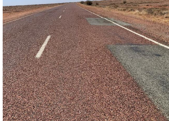
Figure 5.17: Ravelling/fretting – progressive loss of both aggregate and binder from the pavement surface
