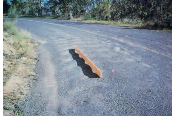
Figure 5.11: Rutting – longitudinal deformation in the wheel path
