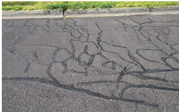
Figure 5.35: Crack sealing
