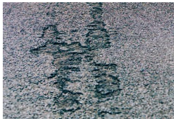
Figure 5.17: Ravelling/fretting – progressive loss of both aggregate and binder from the pavement surface
