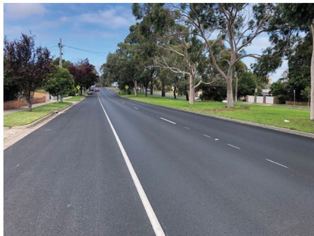
Figure 1: Crumb rubber asphalt at East Boundary Road
