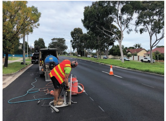
Figure 5: Extracting cores from completed trial sections
