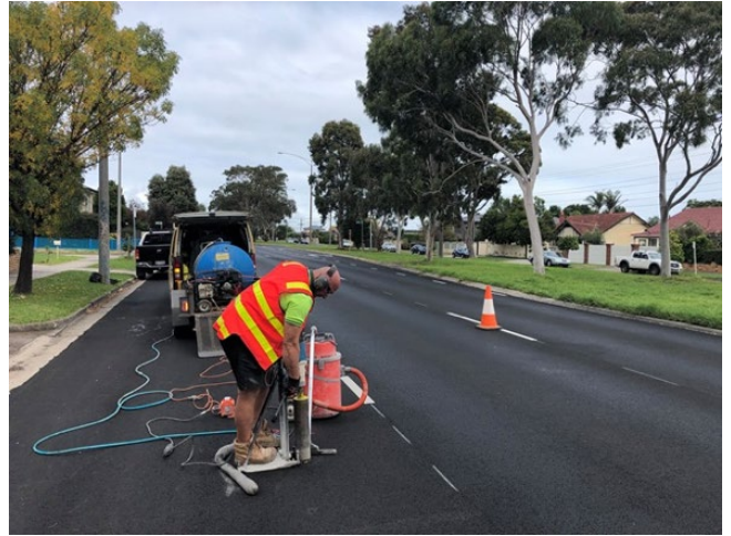
Figure 5: Extracting cores from completed trial sections
