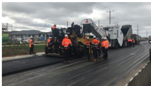
Figure 5: Western Roads Upgrade using recycled materials such as reclaimed asphalt pavement (RAP), crushed concrete and crushed glass
